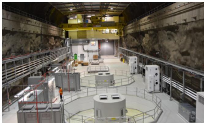
The underground John Hart Generating Station. The generating station's capacity increased by about 10% over the old facility, using the same amount of water. It creates enough power to serve about 80,000 homes.
